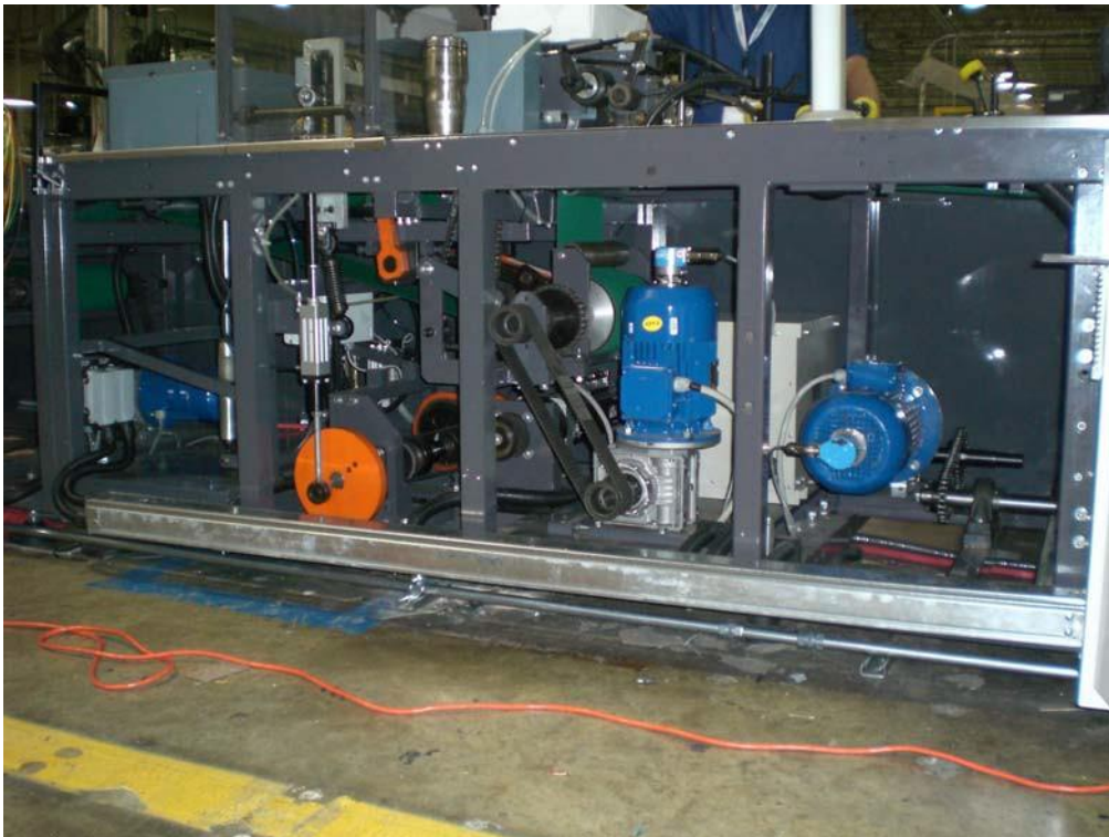
Newly Installed motors With timing belt and new electrical conduit
